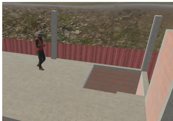
Figure 16: Elevated Work Platform with Void
